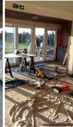
Old Windows removed
