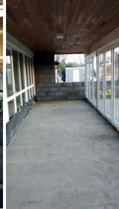
Outside windows in place
