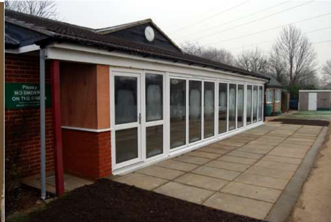
A view of the new doors and glazing
