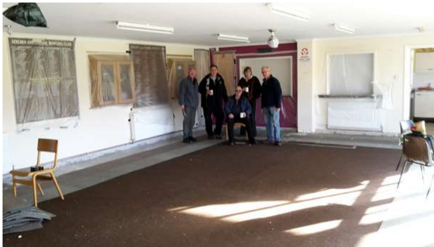
The Clubhouse is cleared, ready for work to commence
