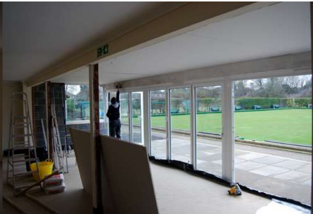
Plaster-boarding in progress in readiness for plastering
