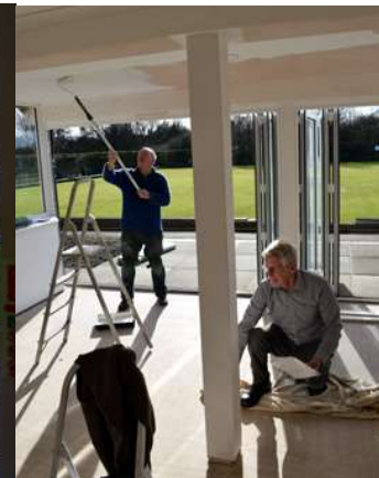
Plastering done, decorating starts
