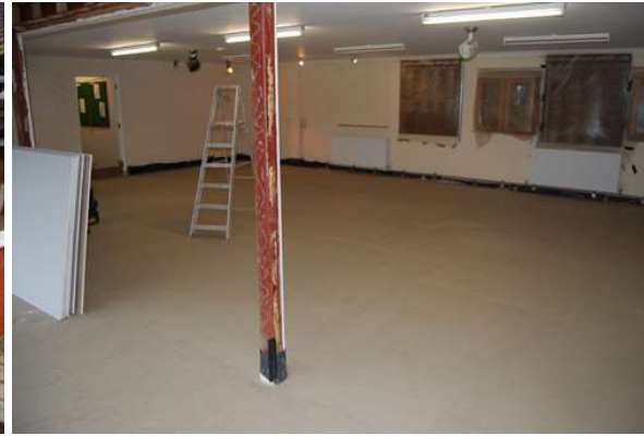
The newly laid, level floor starting to dry.
